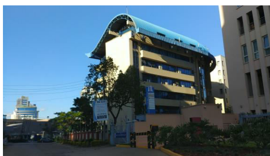
Fig. 26: Shelter Afrique Centre: Mechanical ventilation systems along the western façade
