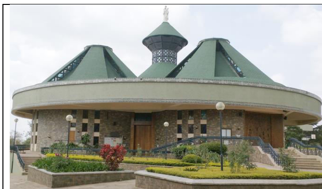
Fig. 23: St. Mary Shrine: Collage of building materials used to achieve tactile, visual and tectonic properties Source: Author 2018
